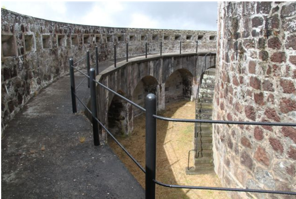
'The Round Tower, showing newly painted railings'
